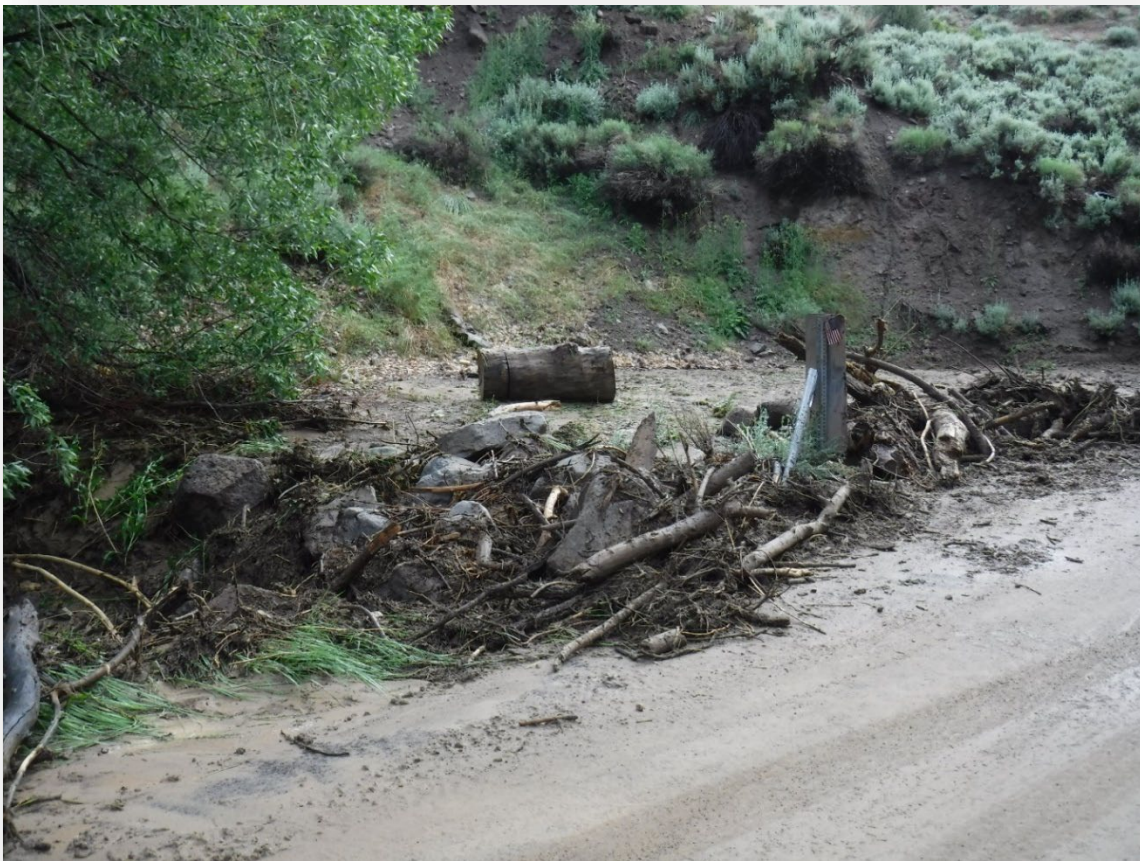
Dead brush, tree branches, and trees washing downstream, further exacerbating the issue.
