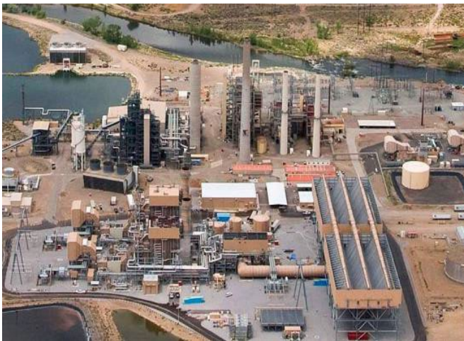
Figure 9.2-3: NV Energy Generating Station Complex at McCarran (Source: NV Energy, 2016)
